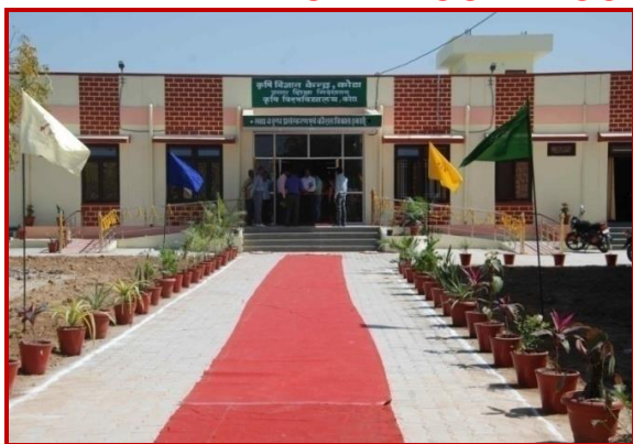
Newly constructed food processing & milk product unit under RKVY
